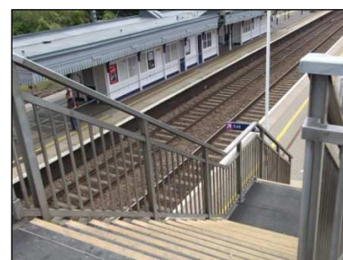
Access to platforms at Biggleswade Station
